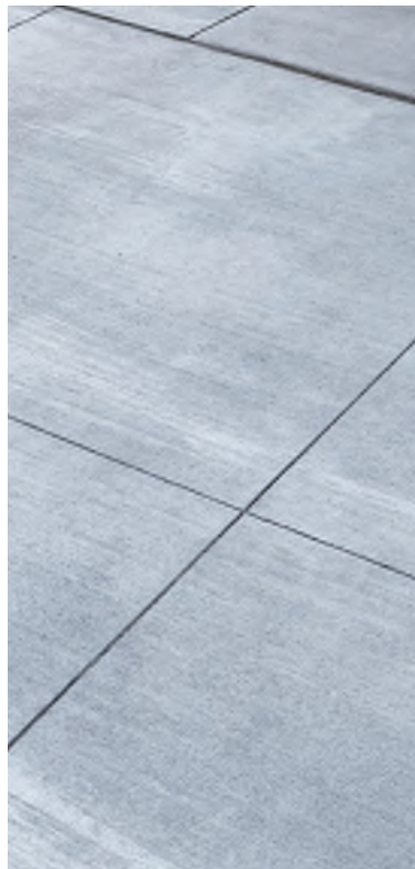
CIP Concrete Paving (Pedestrian & Vehicular) Formal Walkways
